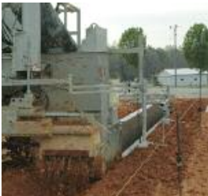
Custom trencher trimmer and poultry house foundation.
