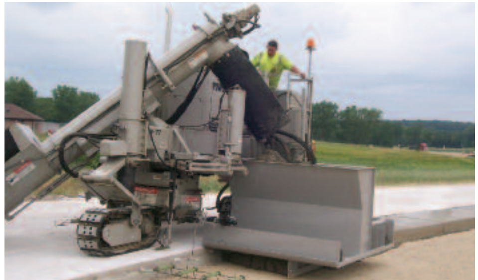
Apron addition over steel, sensing off existing pavement.
