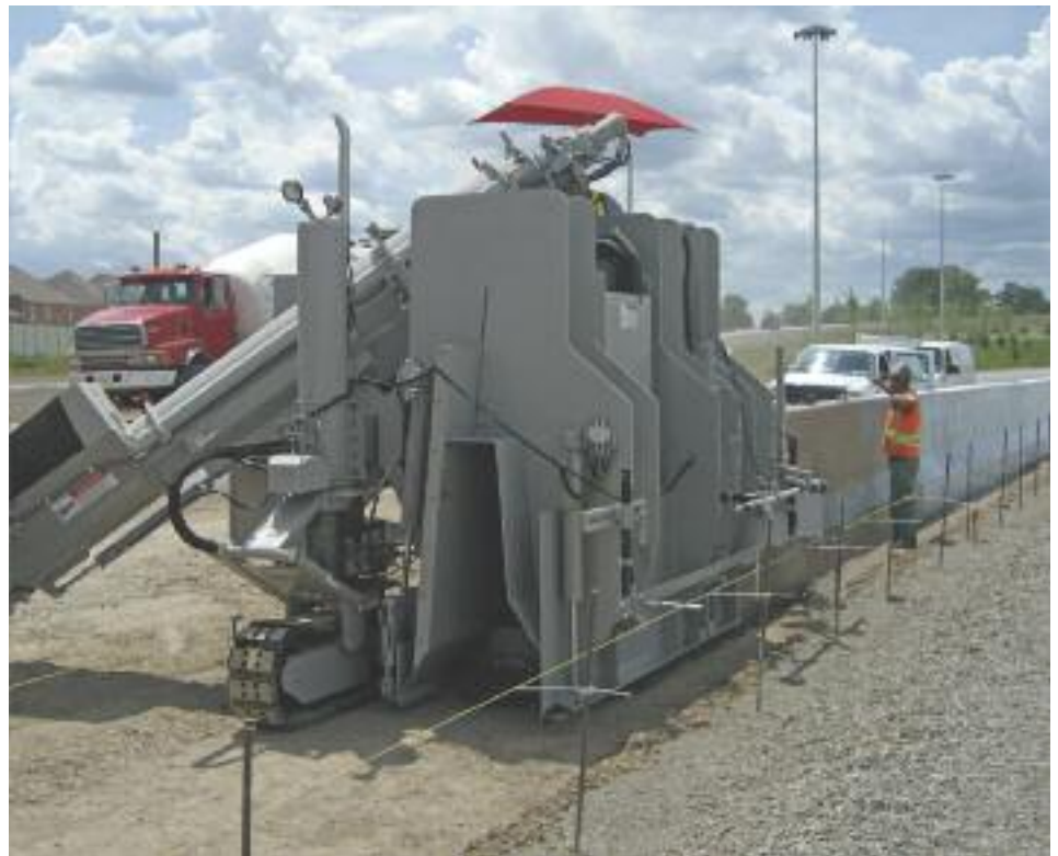
5700-C-MAX pouring large variable barrier wall.
