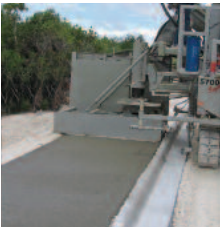
Sidewalk adjacent to back-of-curb. Sensing off-curb.
