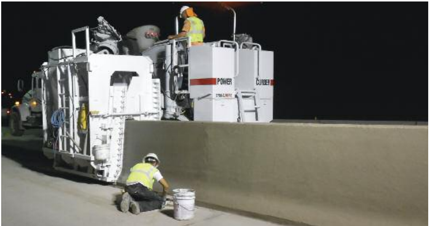
5700-C-MAX pouring at night in Arizona. Variable barrier, from 42" to 56" (1.07 – 1.42m) tall. Optional paint in white.
