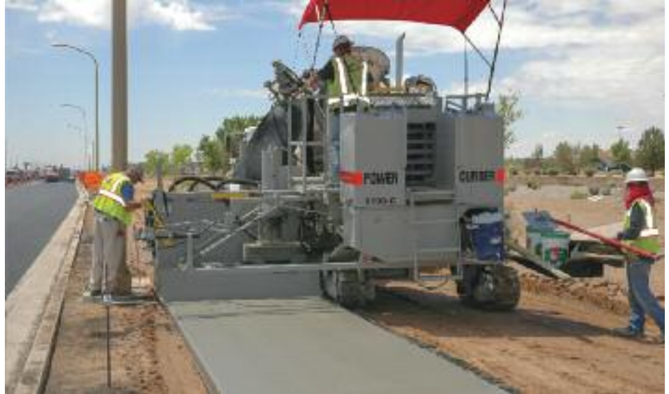
Pouring a 6' sidewalk with minimal side clearance.
