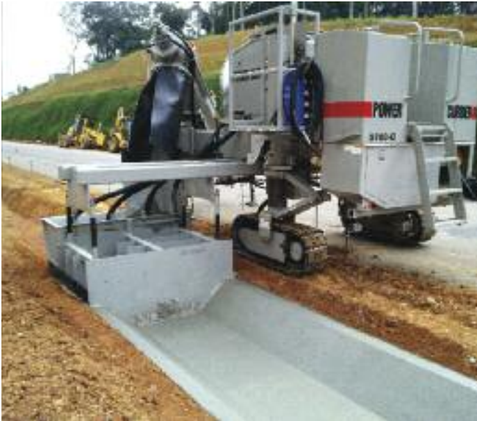
Ditch liner in Equatorial Guinea, 5' (1.5m) wide and 1' (.3m) deep.
