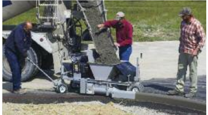
▲ Power Curbers 150 Extruded Curb Machine
