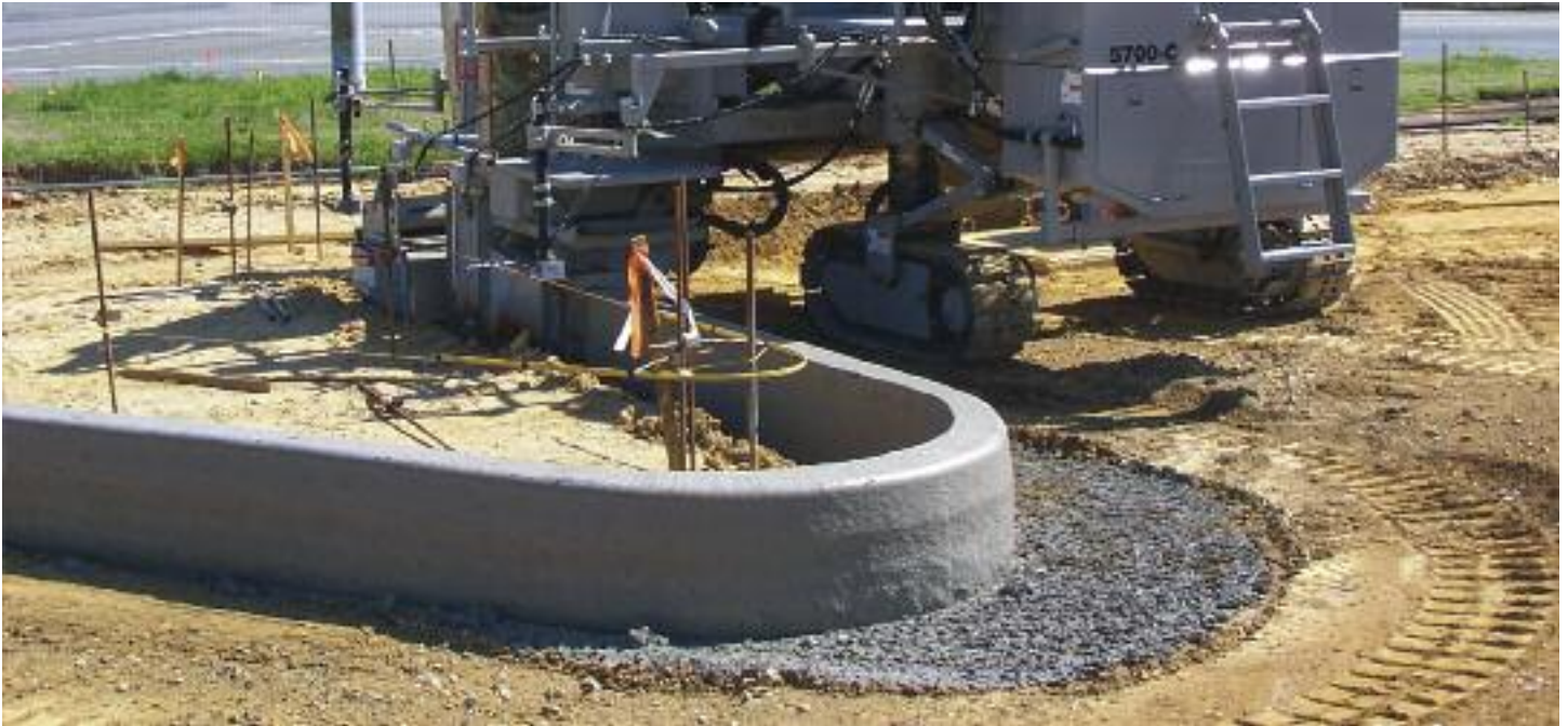
The machine's tight radius capability eliminates hours of hand forming and produces a higher quality product.
