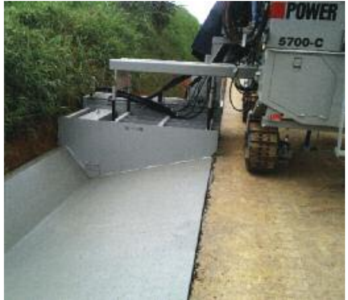
V-Ditch, 7' (2.2m) wide and 18" (.45m) deep, poured adjacent to pavement.
