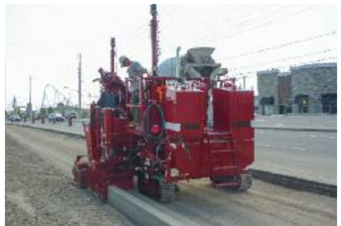
Pouring curb & gutter with 3-D (stringless) control.
