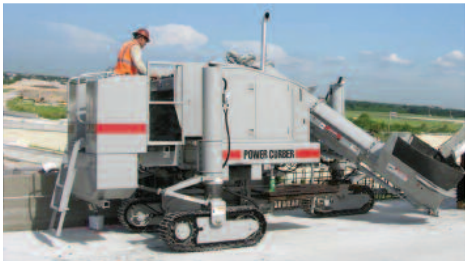
5700-C pouring bridge parapet in Florida.
