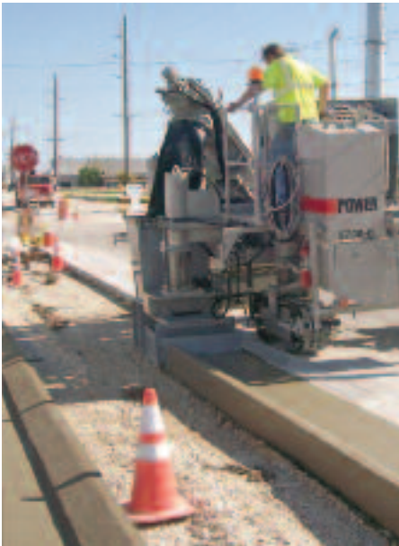
Tapered curb & gutter, poured over dowels adjacent to the pavement.
