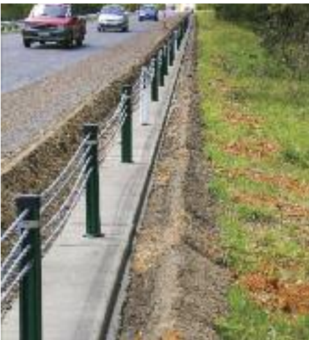
The 5700-C is an all-in-one solution for installing no-mow strips for cable barriers.
