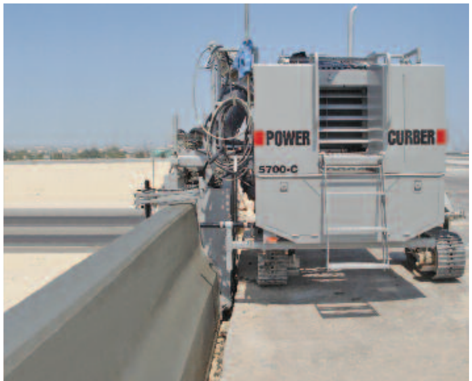
Barrier poured below grade, 49" (1.25m) tall.
