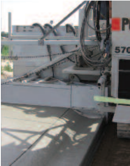
Monolithic curb, gutter, and sidewalk.
