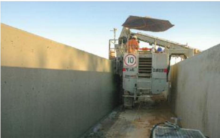
Canal in Australia, base 12' 5.5" (3.8m) wide and sides 6'10" (2.1m) high.
