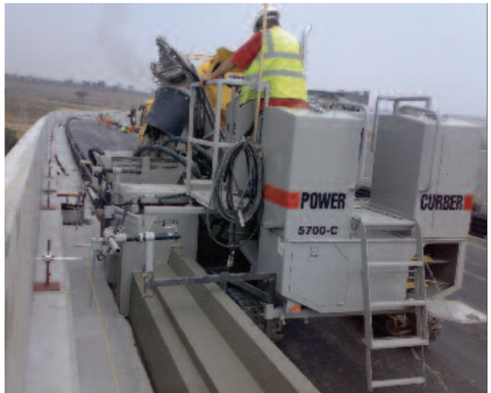
High-speed rail application in South Africa, pouring encasement over electrical conduit.
