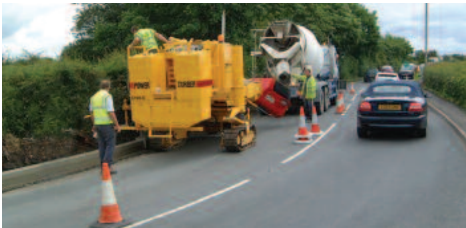
Single-lane pouring minimizes traffic interruption.
